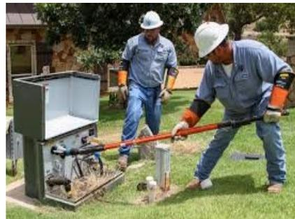
A transformer box is a locked steel cabinet mounted on a concrete pad that contains a securely grounded, energized connection for one or more customers. These transformers are used with underground distribution lines to step down the primary voltage on the line to a lower voltage used in your home.
